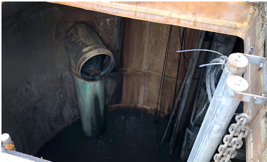
Figure 10. MLS CC6 Influent Drop Pipe
