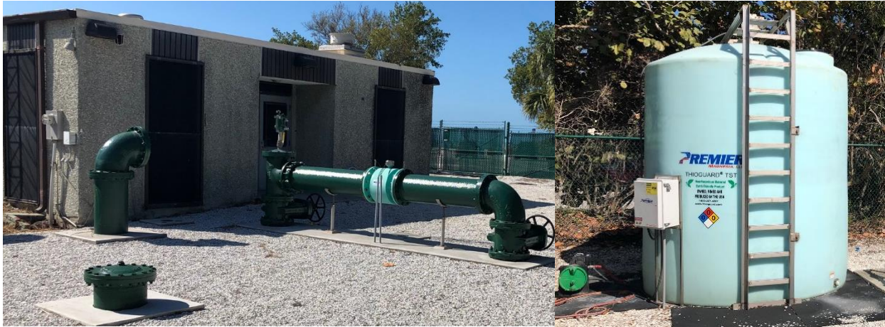
Figure 6. LS 5 and Magnesium Hydroxide Dose System
